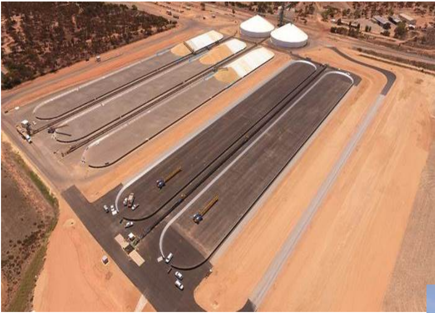
New open bulkheads at Koorda, WA
