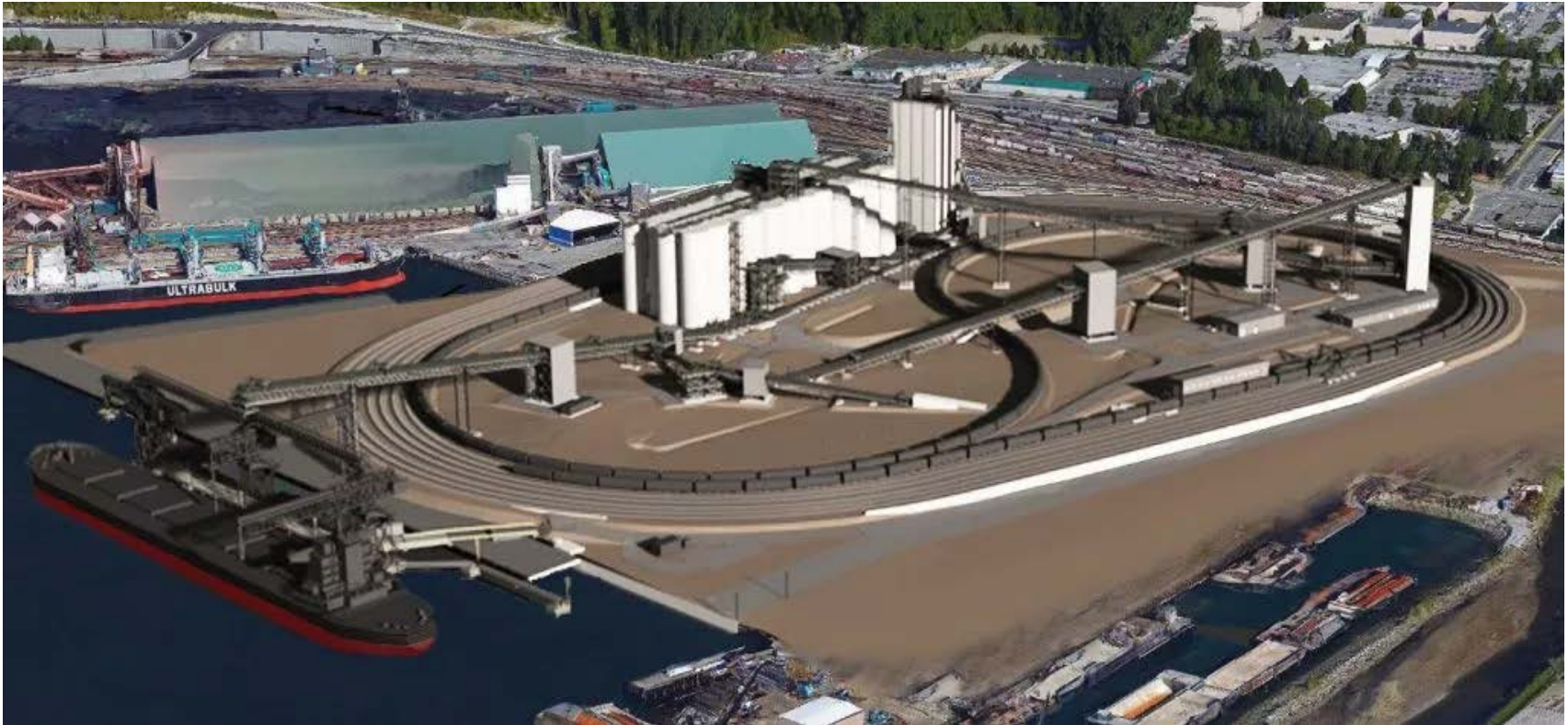
G3 terminal under construction at the Port of Vancouver, Canada (180kt port storage, 6mmt annual export capacity, opening in 2019)
